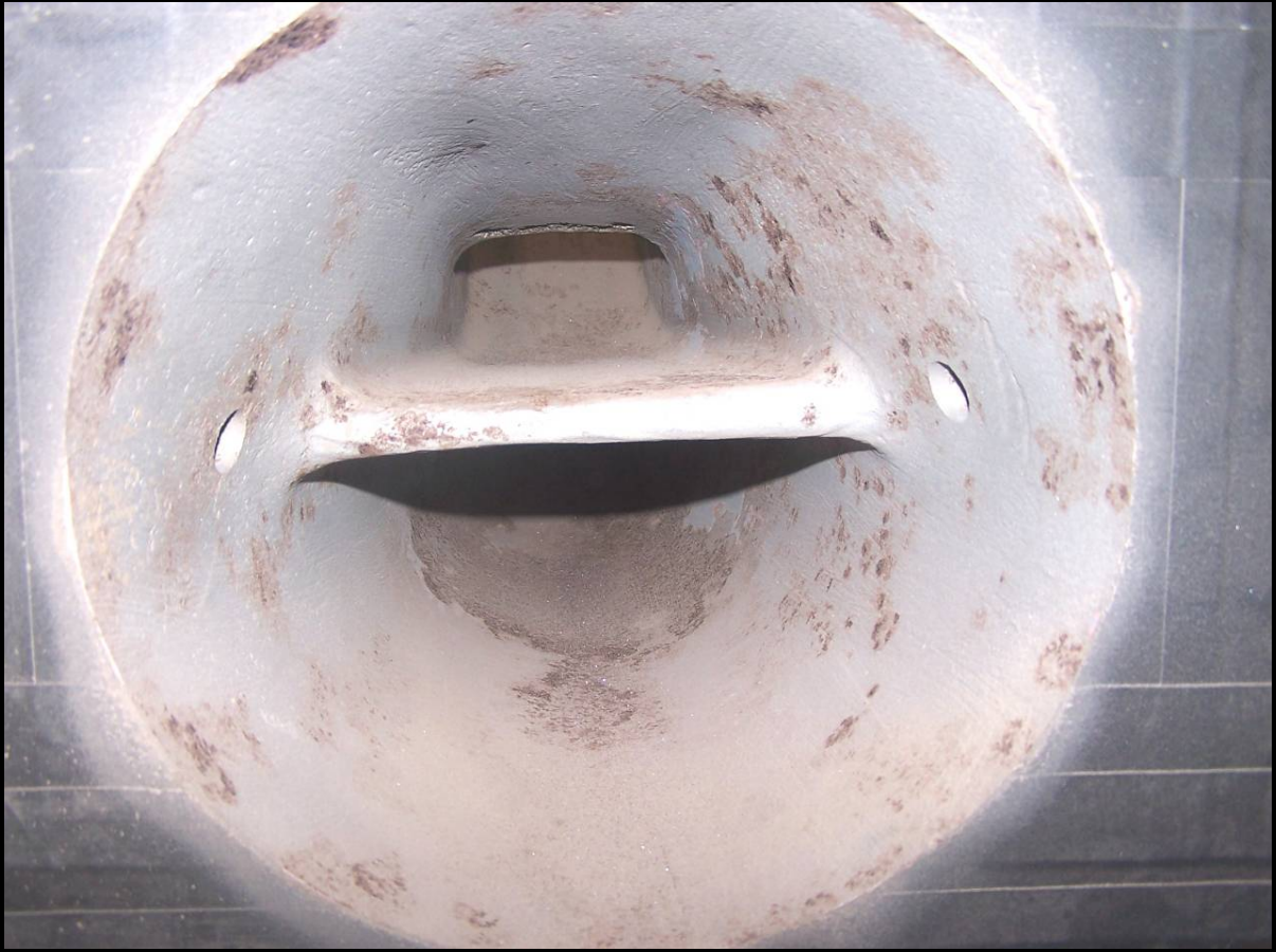
Picture 8 - Original surface coating removed by shot-blasting
