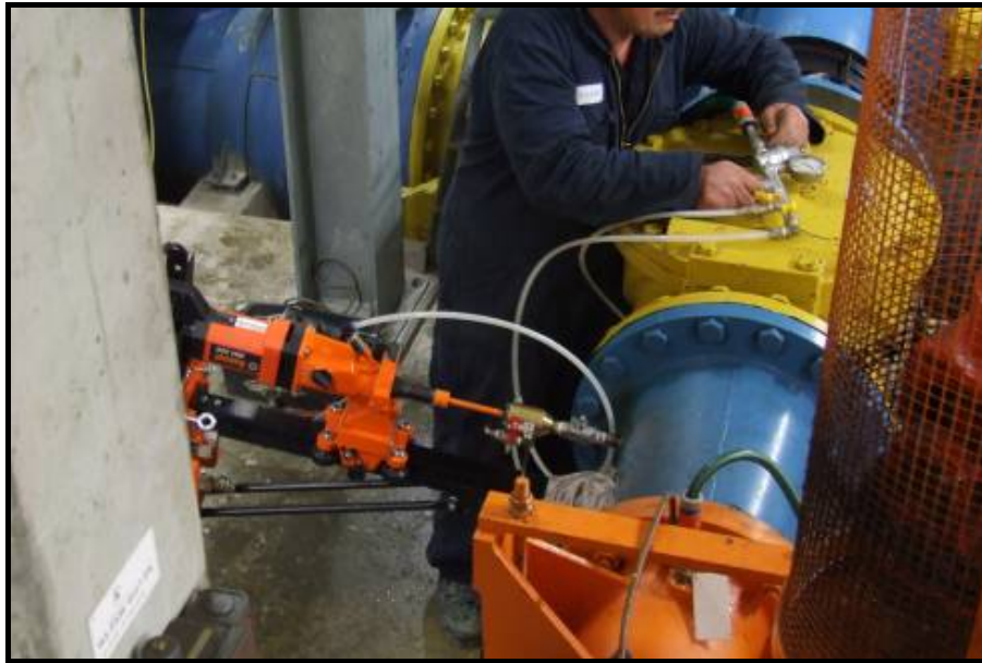
Picture 1 – ‘Hot-tapping’ of pipe
