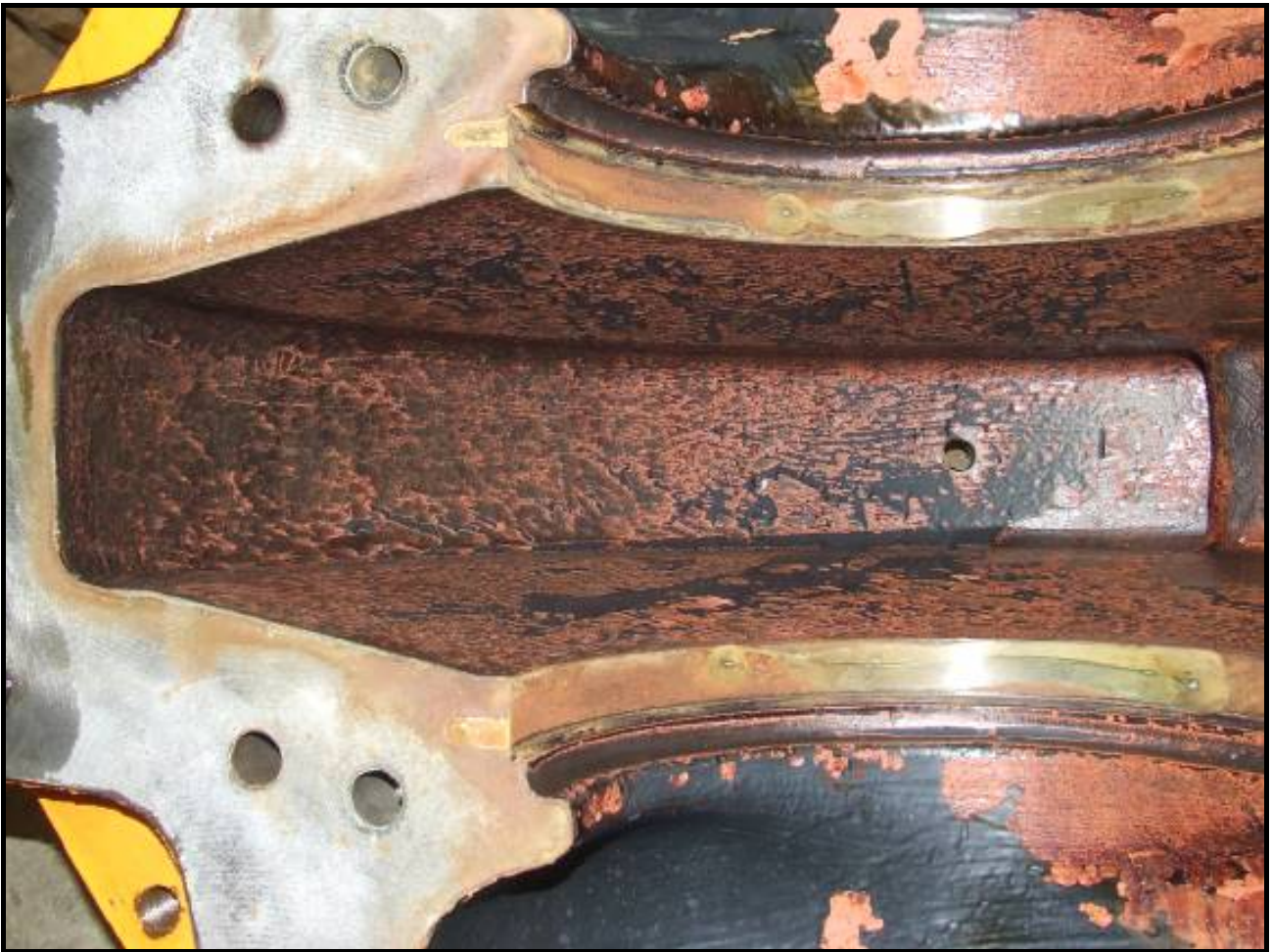
Picture 3 - Surface condition of pump casing after 41,000 hours service
